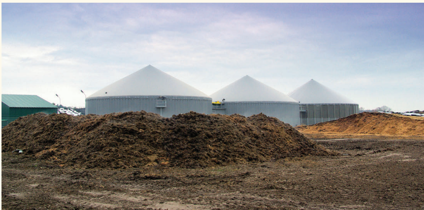
Biogas Plant • Credit: LianeM, Shutterstock
